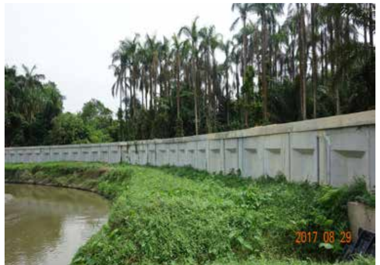
Slope and Bank Stabilization Drain, Canal, Pond, Lake and River
