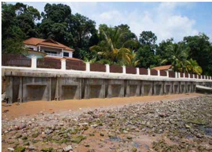
Marine Structure Wharf, Jetty, Coastal Protection
