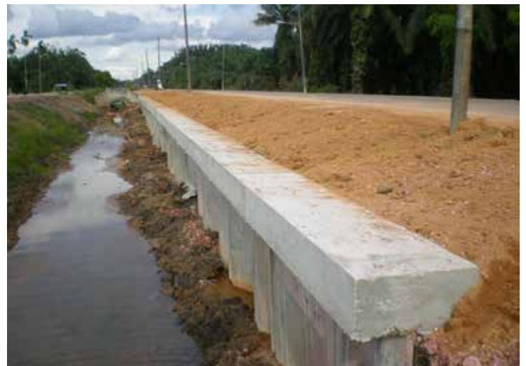
Roadwork Embankment, Bridge, Abutment and Wingwall
