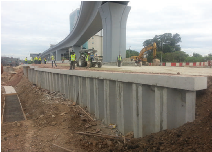
Roadwork Embankment, Bridge, Abutment and Wingwall
